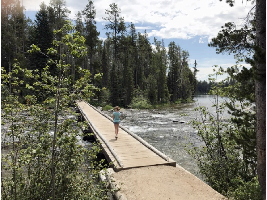
Leigh Lake Outlet Bridge
